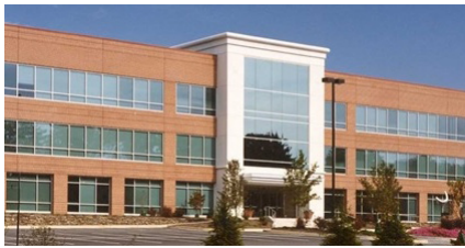
NEW Maryland Office
